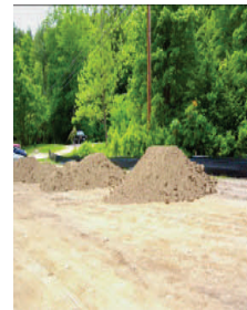
Ground breaking work begins at Hartshorne Pond. (Rt 13N)
